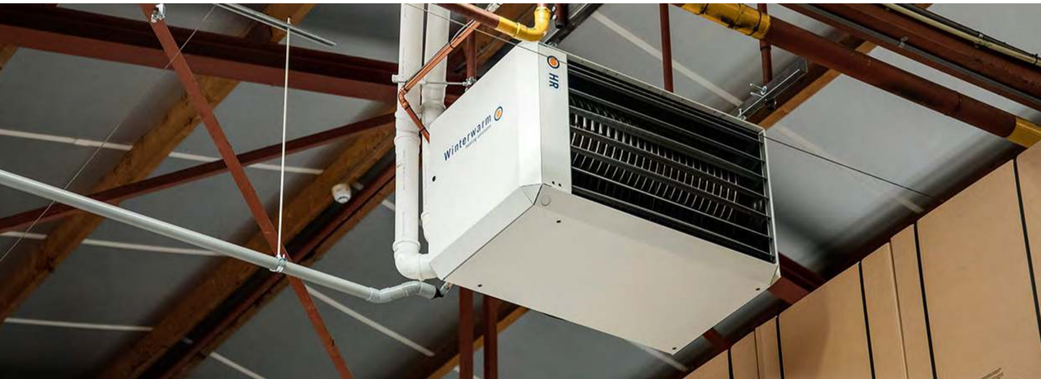
Afb. 7. HR-gasheater (foto Winterwarm Heating Solutions)
